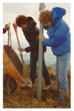
Upon completion of the four foot deep hole, Richard ZL2UGC holds the bottom section of the mast while Michael ZL2TDT pours the concrete.
