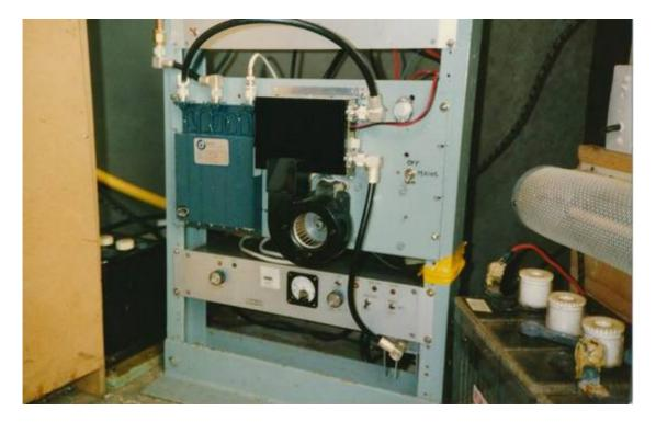
You can see that the Pye U450L unit was replaced, DC power supply and PA duplexer retained and the controller now fitted at the top of the rack.
