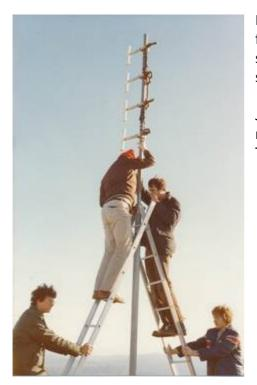
The completed installation. Power was measured at dipoles as 15 watts feeder loss 0.54db. First contacts Jeff ZL2CW and Gretta ZL2AGS. Then John ZL2TRV (ZL4RF) spoke to Ralph ZL1TBG in Walkworth north of Auckland. The machine worked well.
